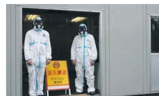
An Industry-first Asbestos Treatment Facility
